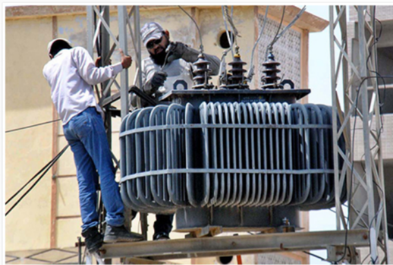
Installation of PMT
